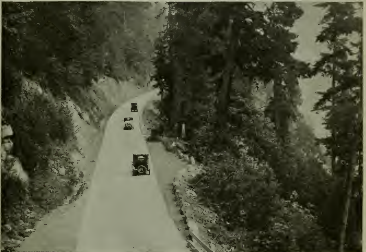
Thousands of miles of concrete roads have been laid in the United States and Canada. In the United States alone enough has been laid to make twelve roads from the Atlantic to the Pacific. This is a bit of the Chuckanuck Drive near Bellingham, Washington, and is a part of the Pacific Highway.
